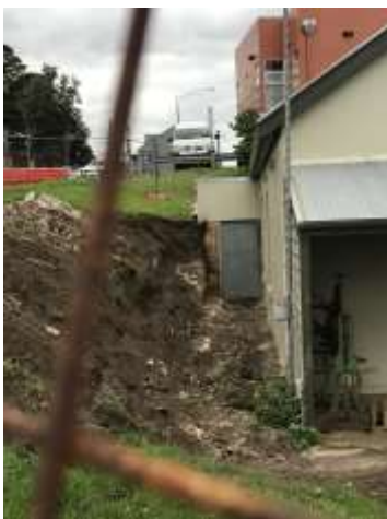
Excavation work to rebuild sandstone wall at History House
